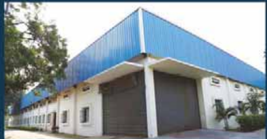
Hydraulic Valves Plant
