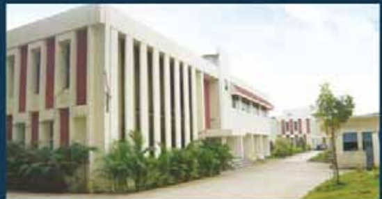
Gear Pumps Plant
